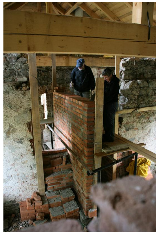
The Mauricovna was reroofed and internally reconfigured
